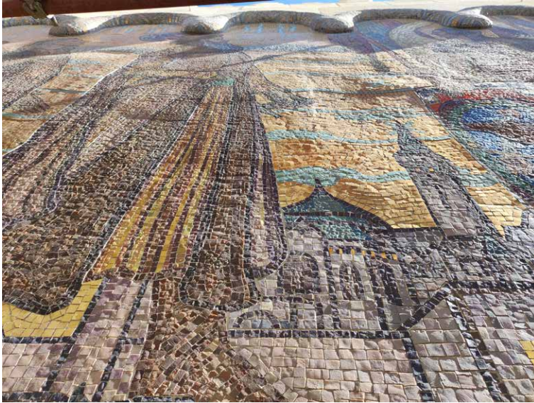
Fig. 1. Detail of the mosaic "Patrona Hungariae" of Aladár Körösfői-Kriesch and Miksa Róth (1913) on the main façade of the Culture Palace in Marosvásárhely/Tg. Mures. In raking light the original uneven surface character of the mosaic is well visible. The phenomenon is resulted from the mounting process of the prefabricated sections.
