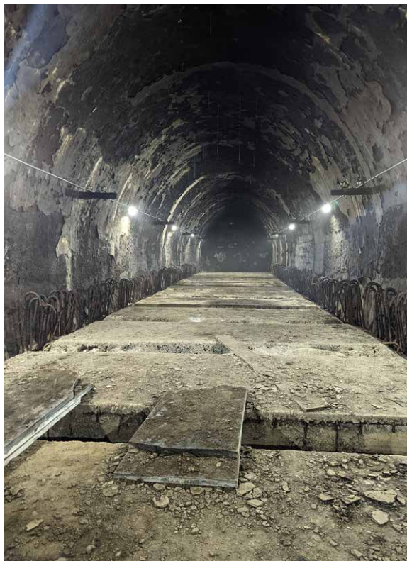
Fig. 2. Tunnel where mosaics were stored. (Photo: M. Protić)
