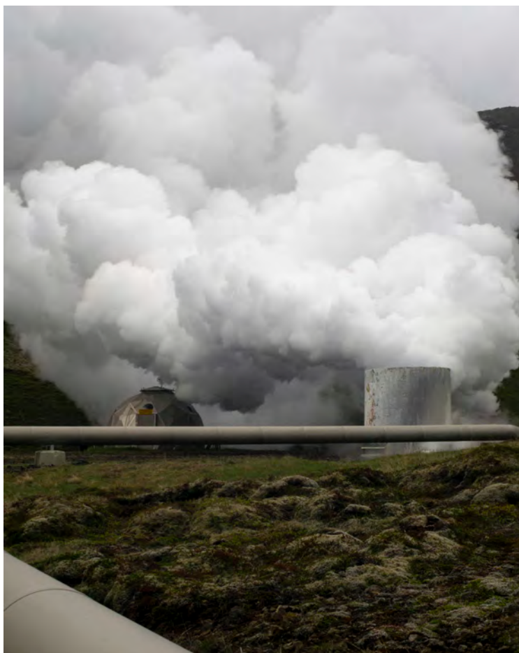
Fig. 5.: Untitled, borehole and pipes near Nesjavallavir geothermal power plant, digital photograph, 2024
